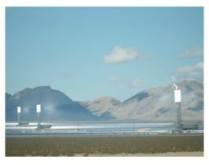
about 9 m tall and 24 m in diameter. Molten salt is used in solar power tower systems because it is liquid at atmospheric pressure, has operating temperatures compatible with modern steam turbines, is low-cost, and is non-flammable and non-toxic.
